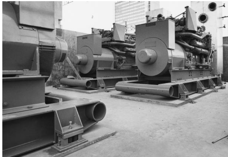
CAT. D399 Generator sits on LO-REZ LR4-LS Isolators. Westcoast Transmission Building, Vancouver
